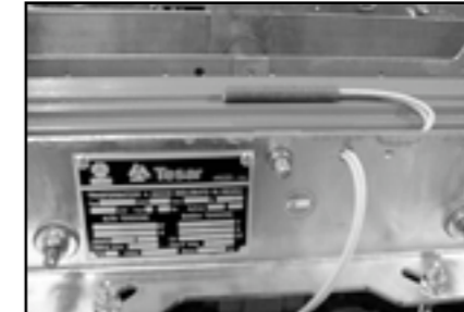
Fig. 4 Double PT100 on the core
