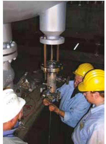
Installation of a multi-point thermocouple
